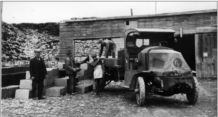
Three men load pallets of slate onto a large truck at the Big Boy Quarry, owned by Hugh G. Williams. The gentleman posing with them in the slate yard is Thomas Barrington Sr., quarry superintendent. Photograph dates to about 1920.
